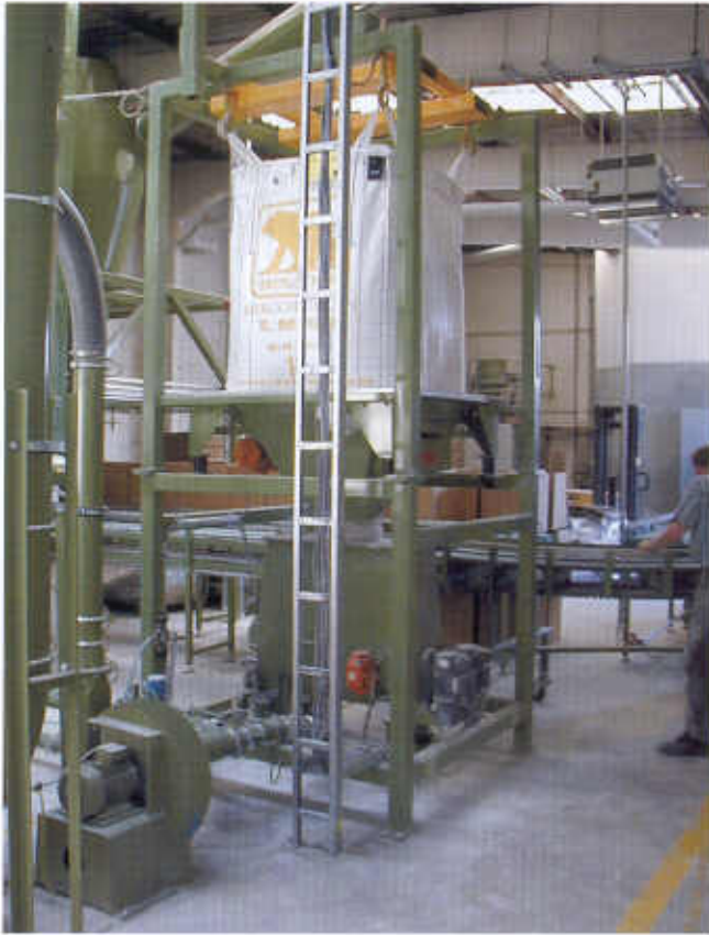
Dusting agent installation
